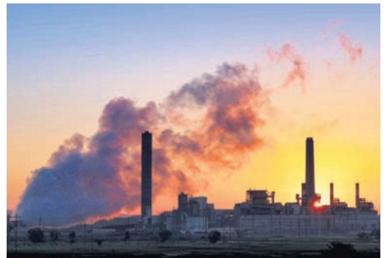
In this July 27, 2018, file photo, the Dave Johnson coal-fired power plant is silhouetted against the morning sun in Glenrock, Wyo.
